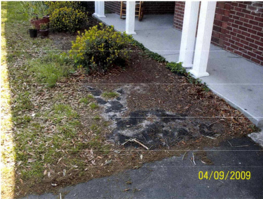
Picture 1: UST 279Birch excavation site prior to removal.
