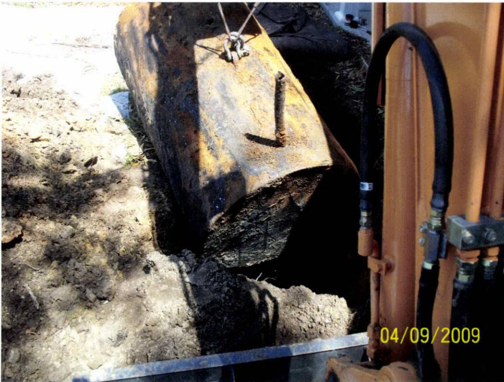
Picture 2: UST 279Birch immediately after removal from excavation.
